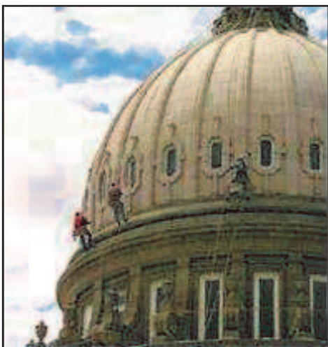
Idaho capitol dome, upper lantern masonry, and terra cotta repair work was completed in 2005.
