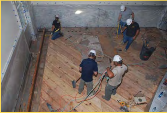
Construction workers remove sections of the fourth floor that had been added to create additional space.
