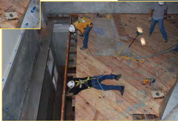
Construction workers remove sections of the fourth floor that had been added to create additional space.
